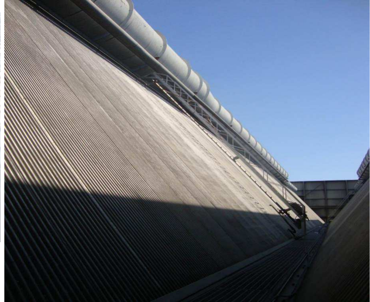
Tube Bundle System (A-Frame)
